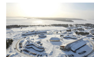
Aerial view of Oujé-Bougoumou town centre (Tourism Office/Post Office, Chiisemandoo-Miichwahp, Nation Headquarters, and Aanischaumkamikw Cree Cultural Institute). Image source: Projets Verts
